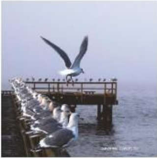
Davis Bay Pier 1
