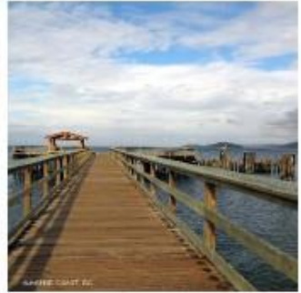
Davis Bay Pier 2
